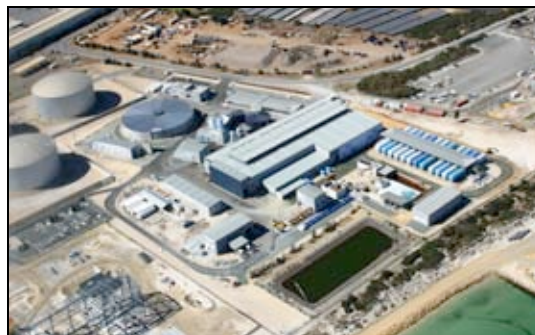
Figure 2: Perth Seawater Desalination Site – March 2007
