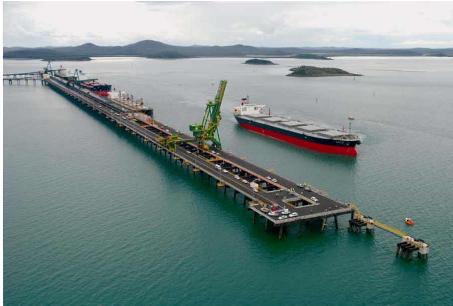
Figure 5 - Completed Berth 4 and Associated Works
