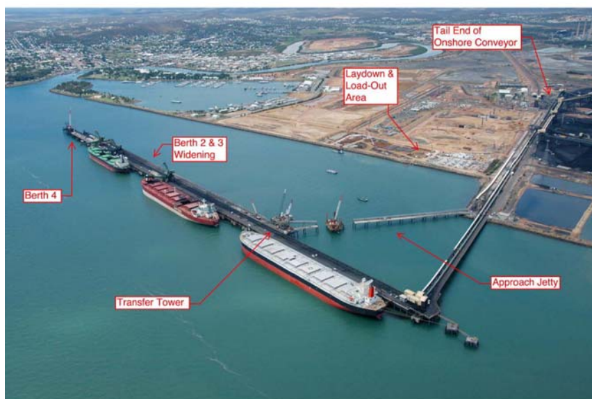
Figure 1 - Works at RG Tanna Coal Terminal
