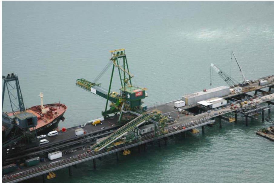
Figure 4 - Shiploader 3 on the end of Berth 3, Berth 4 Works Underway
