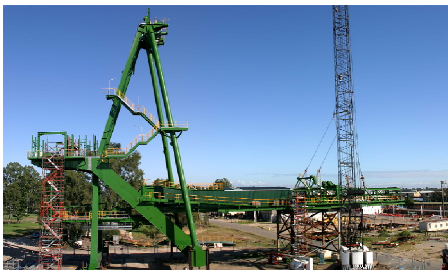
Figure 2 - Shiploader 3 assembly in Brisbane
